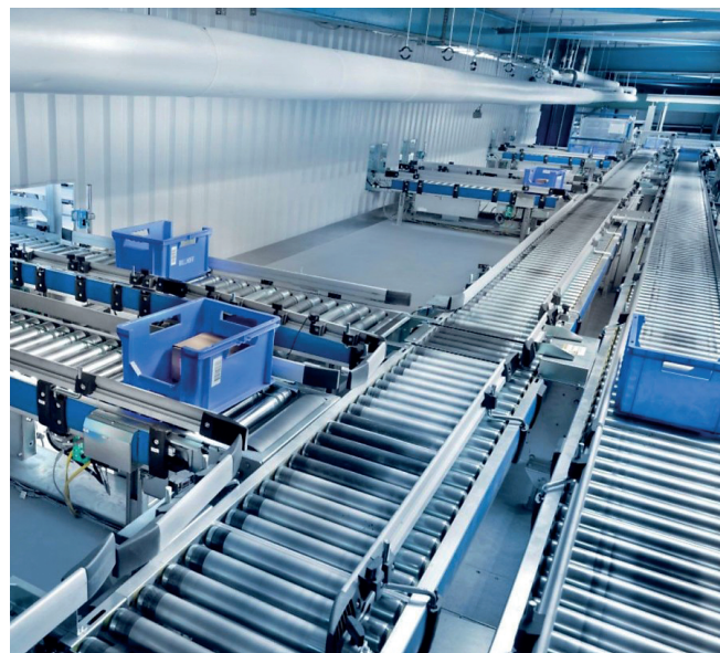
Secondary Battery & 일반물류 Conveyor
